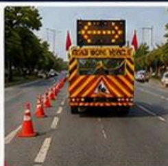
WORK ZONE SETUP
